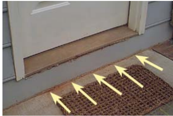
Caulking gaps between porch and siding helps.
