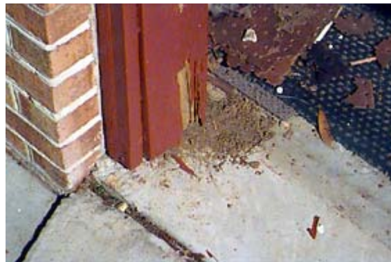
Probe wood to check for decay or termites.
